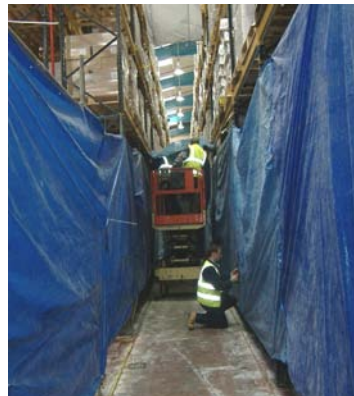
Rigging the tent
