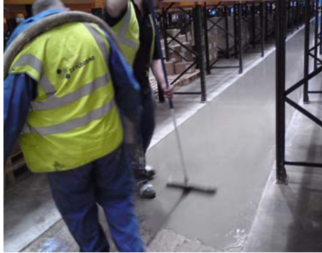
Application of FASTFLOOR - IT
