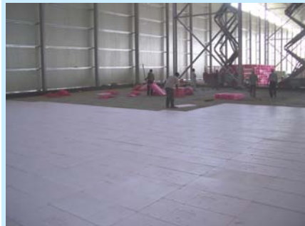
Under slab insulation being placed in preparation of casting
