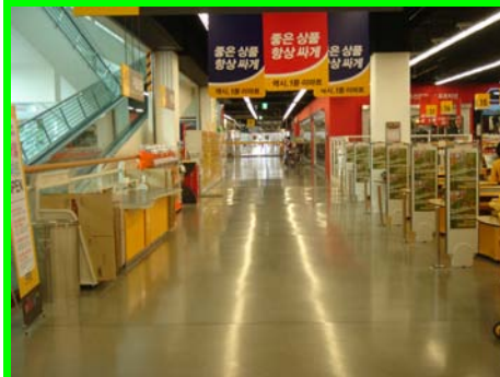
Completed Concrete Topping Floor at E-Mart Hypermarket
