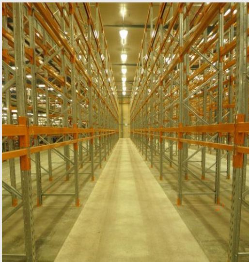
Ground narrow aisle using the Laser Grinder®
