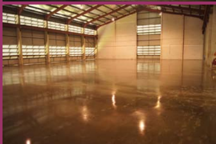
Photos from left: Rebar panel installation completed; High quality FM3 flooring
