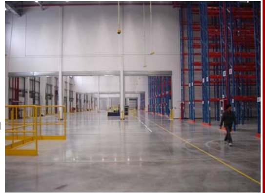
Top: Jiashan DC. Below: Construction in progress
