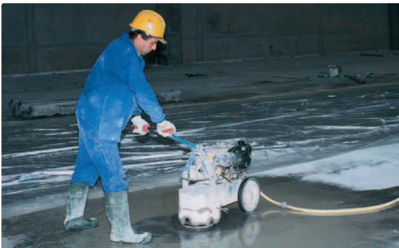
Figure 1: Walk-behind manual grinding.
