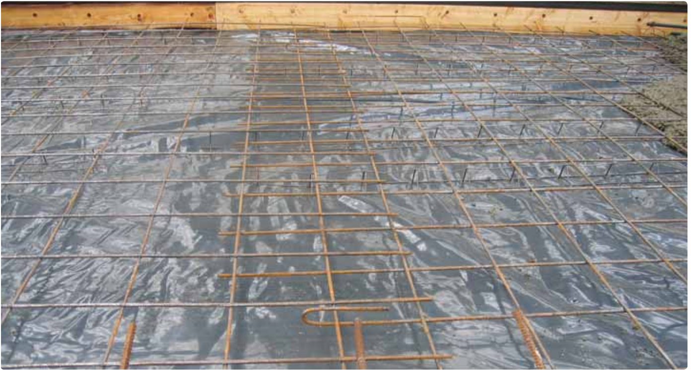
Figure 1: Steel fabric placing.
